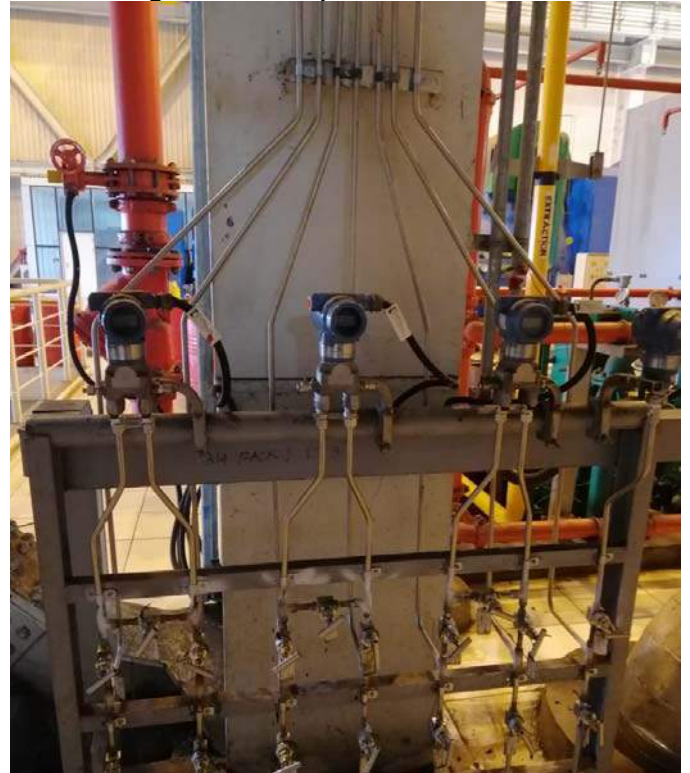
Tubing Installation pada Transmitter Steam
